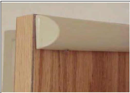
Figure 3.2.6.2: Door Top Pressure Sensitive Alarm
