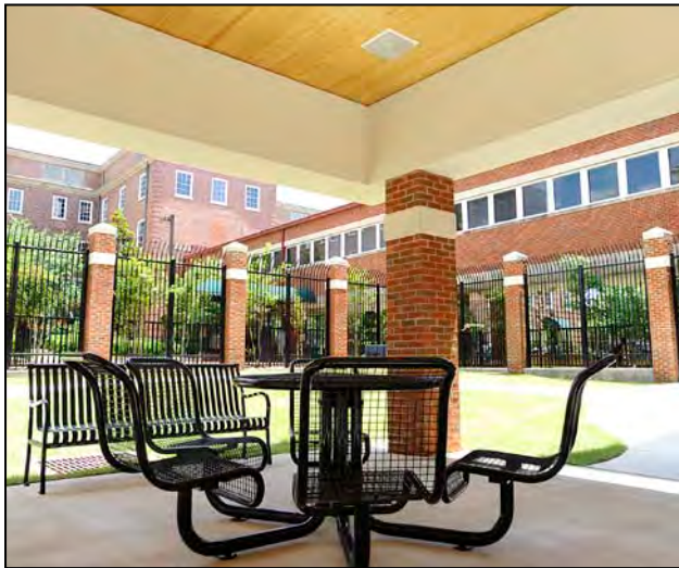
Figure 3.2.9.1: Enclosed Courtyard Example – VA Tuscaloosa, AL
