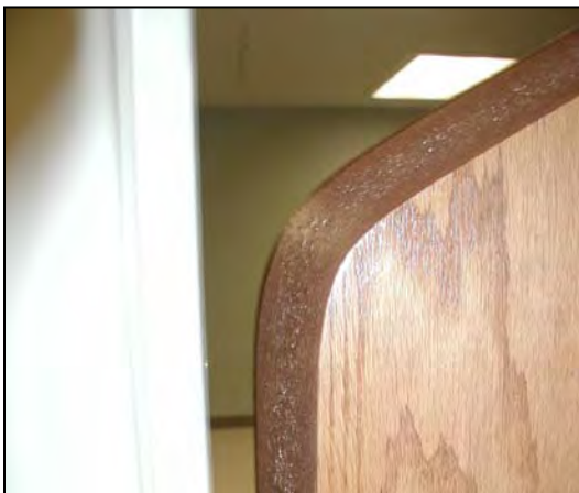
Figure 3.2.6.5: Sloped Patient Door Detail
