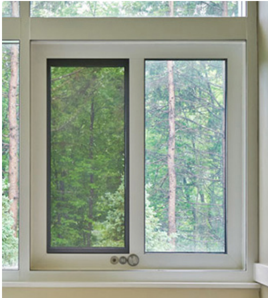
View from Interior - Screen on left panel
